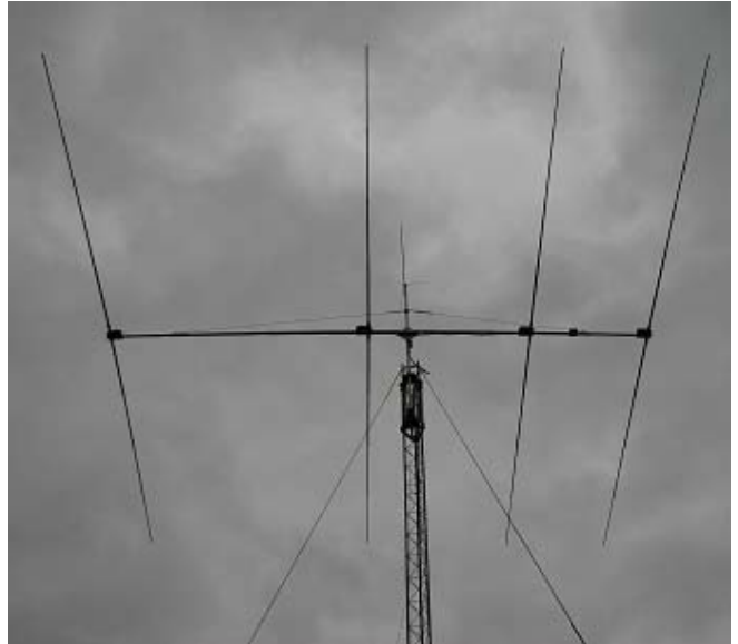
K3SUE's SteppIR 4 element, HF/VHF yagi antenna
